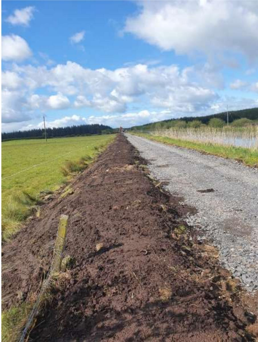
Fig2 – Taken at CH9200 looking South. Embankment, excavation terram & stone base laid.
